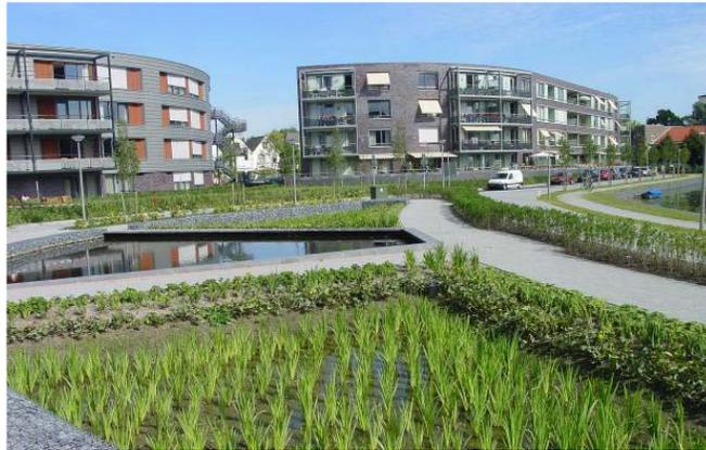
**Figure 5. Example of sustainable drainage systems retrofitted into the urban environment in Holland [11]**
