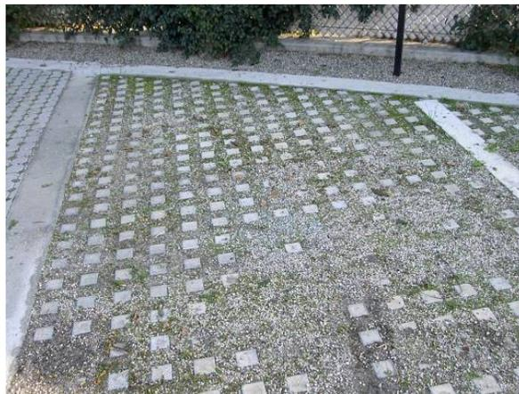
**Figure 3. Porous pavement testing in a parking lot**
