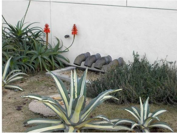
**Figure 2. Example of roof runoff management and impermeable surfaces disconnection**
