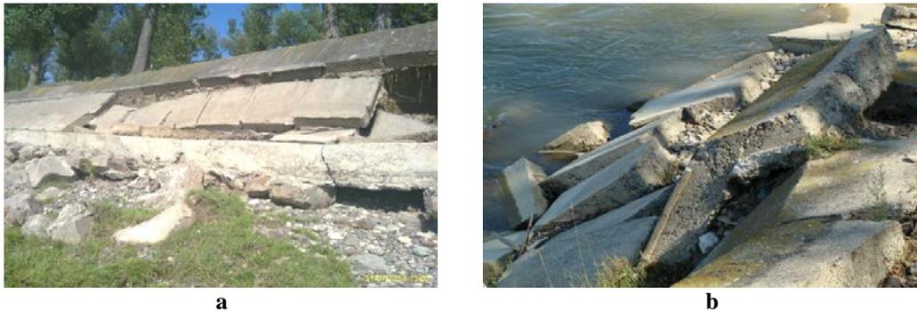
**Figure 6. The condition of shore protection works in Moldova River undercrossing area: a – left shore protection works general view; b – detail on the condition of the concrete slab revetment.**
